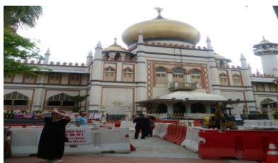
Sultan Mosque, the congregation point; and The Muscat Street Project in progress
