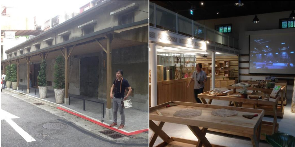
Photo1, 2: Façade and 1st floor of “No.1 granary”
